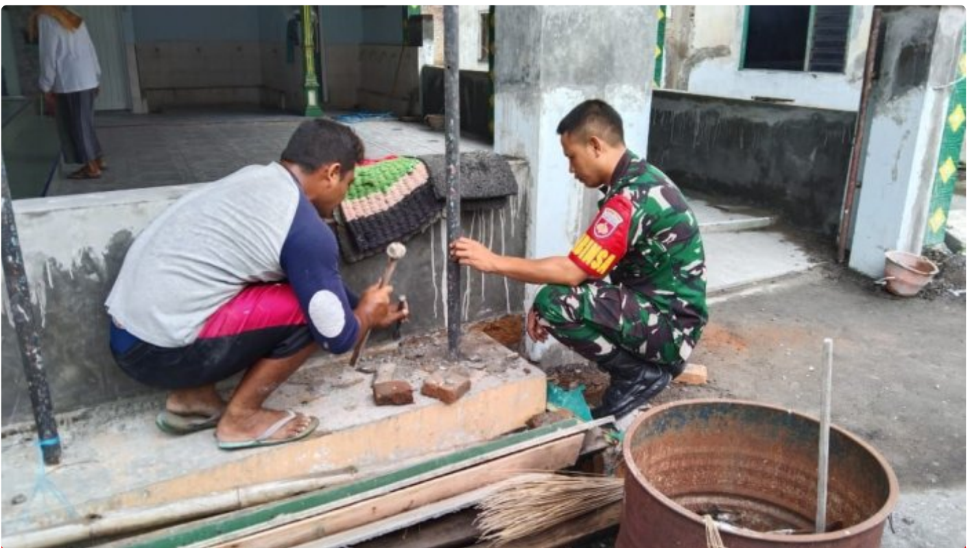
Babinsa Ceper Monitoring Rehab Masjid Di Dukuh Pason
